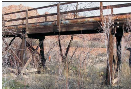
Trestle bearing a pipeline from the river pump station was demolished and will be replaced with an underground pipeline.
