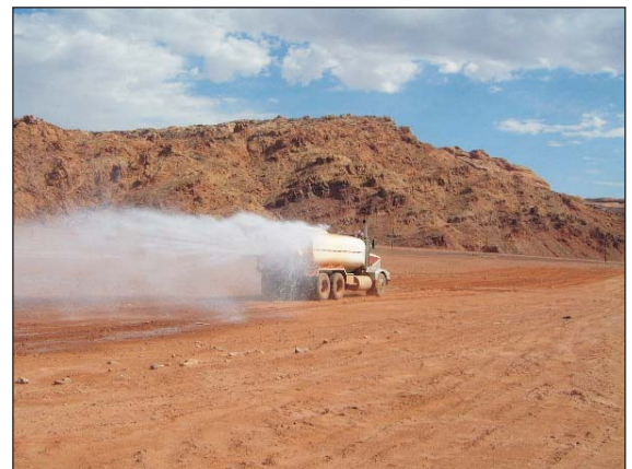
Calcium chloride is applied at the project site to control fugitive dust.
