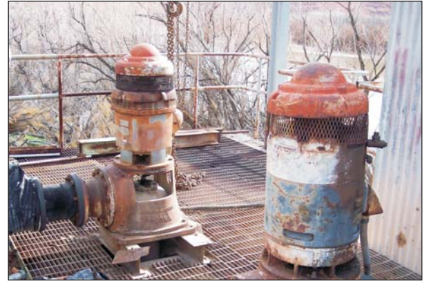
These river pumps will be replaced with more energy-efficient pumps.
