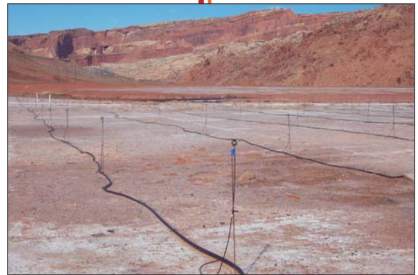
Interim remedial action sprinkler system in operation on top of tailings pile.
