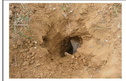
c.) To repair these broken wells we cut the PVS pipe flush and add PVC pipe above the ground surface. We then add a protective steel casing and secure the well with a concrete pad.
