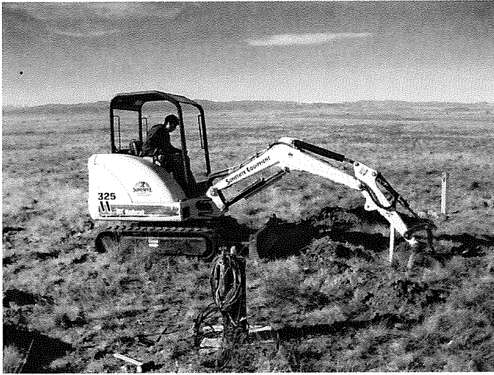
Photo 3 (below): 3/8" sodium bentonite chips are gravity fed into the casing, using a 1/4" screen, to minimize fines from entering the casing.
