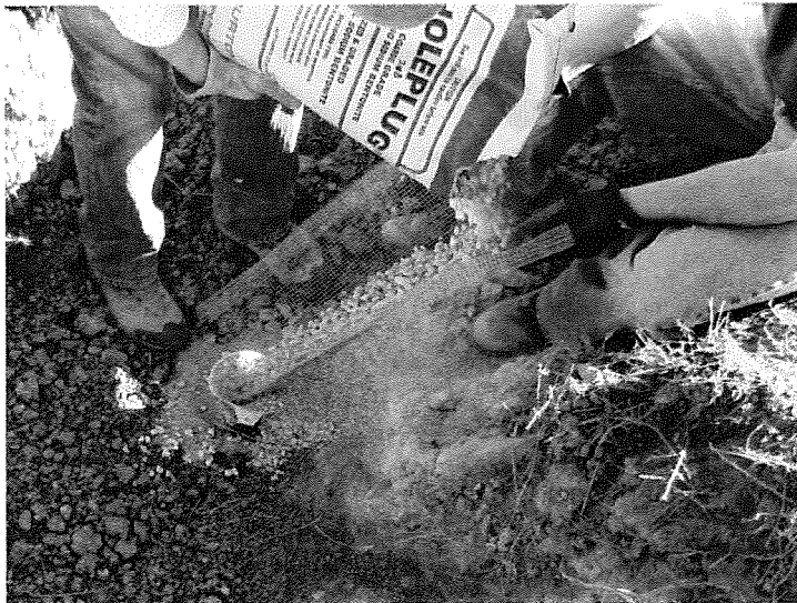
Photo 3 (below): 3/8" sodium bentonite chips are gravity fed into the casing, using a 1/4" screen, to minimize fines from entering the casing.
