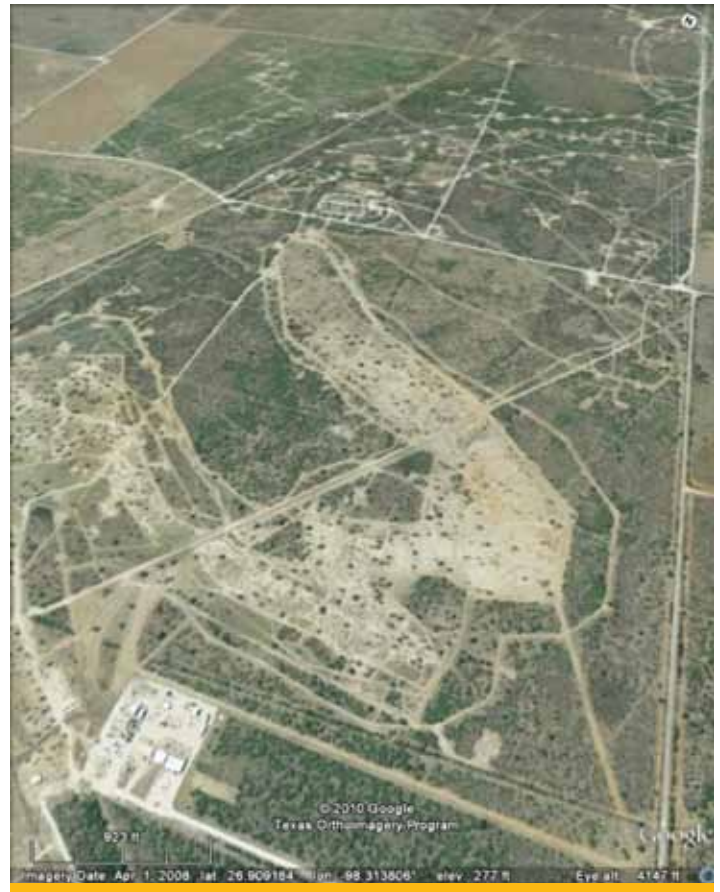
Figure 18: A portion of Mestena Uranium's Alta Mesa in-situ leach facility in Brooks County, Texas. The processing plant is at lower left. Source: Google Earth.
