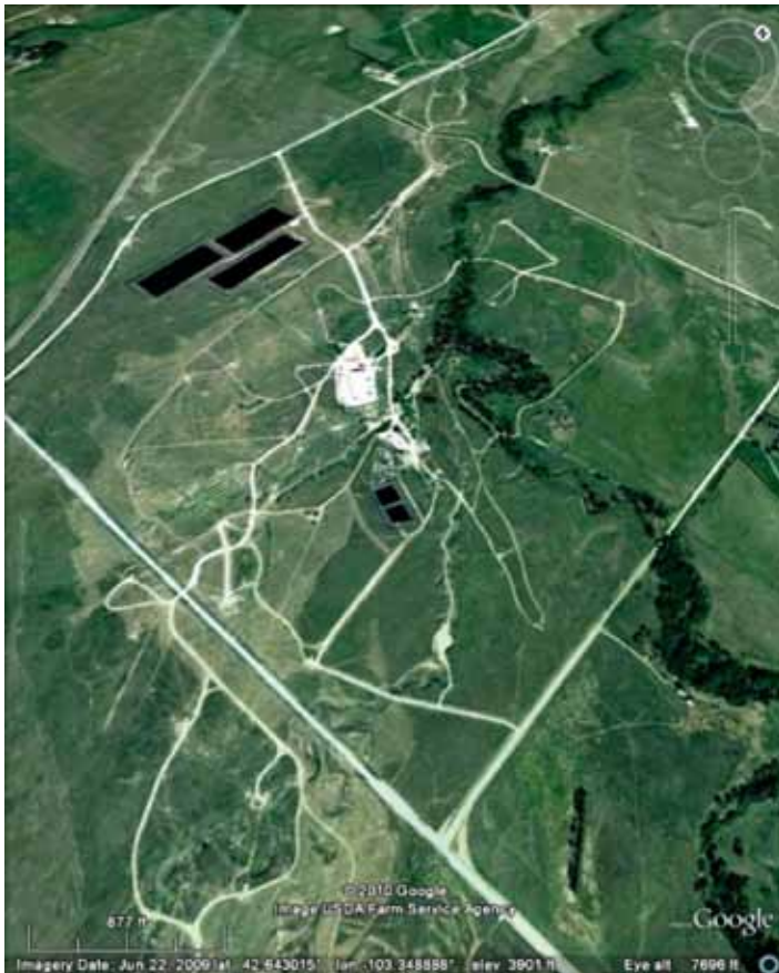
Figure 15: Overview of a portion of Cameco’s Crow Butte uranium in-situ leach facility in Dawes County, Nebraska. Source: Google Earth.
