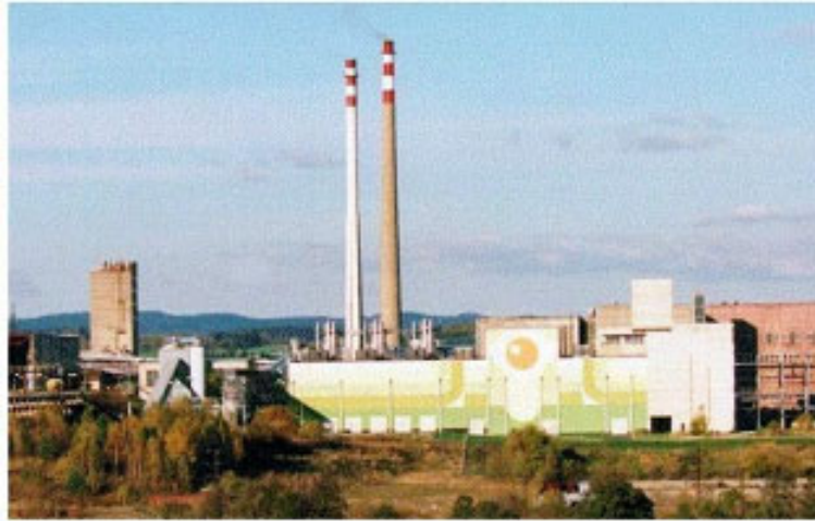
FIG. 40. Evaporators and crystallizers building (Desalination plant stage I).
