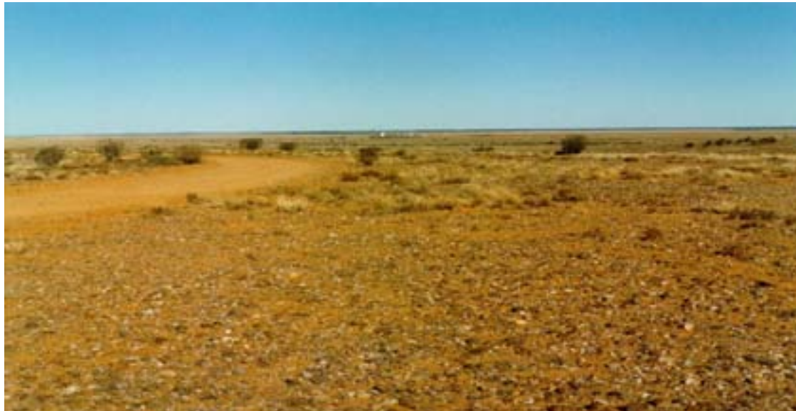
FIG. 10. Existing plant viewed from mine access track.
